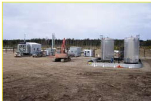
Saxon Compression and Dehydration Facility in final stage of construction
